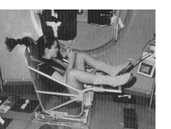
Figure 1.2.9 Newton's first law in action. It is important to know about changes in body mass of astronauts during long periods in orbit. Obviously bathroom scales are useless in this situation. This device uses the inertia of the astronaut's body to affect the way in which oscillations happen – the oscillations are then timed and used to calculate the mass of the astronaut.
